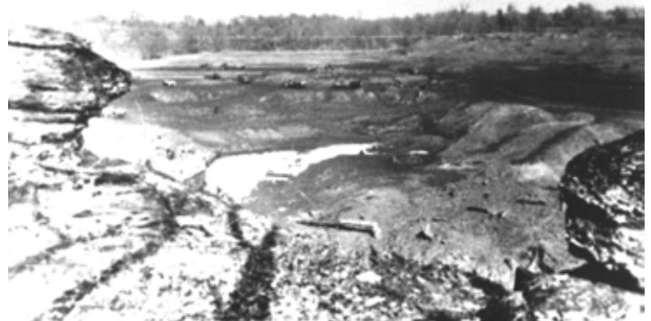
Under construction, 1927. Dam and railroad in background.
